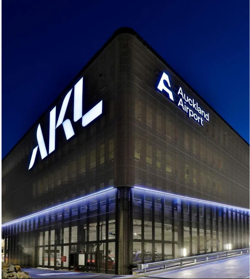
Achieving improved financial performance while fostering a dynamic commercial precinct that drives prosperity for New Zealand through tourism, trade, and enterprise
