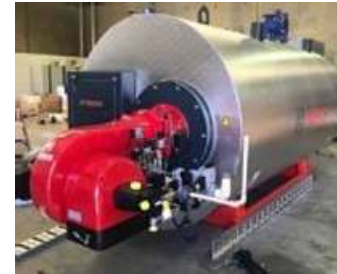
Industrial Package Boiler
