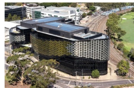
Building 3, 570 Swan Street, Richmond, Victoria
