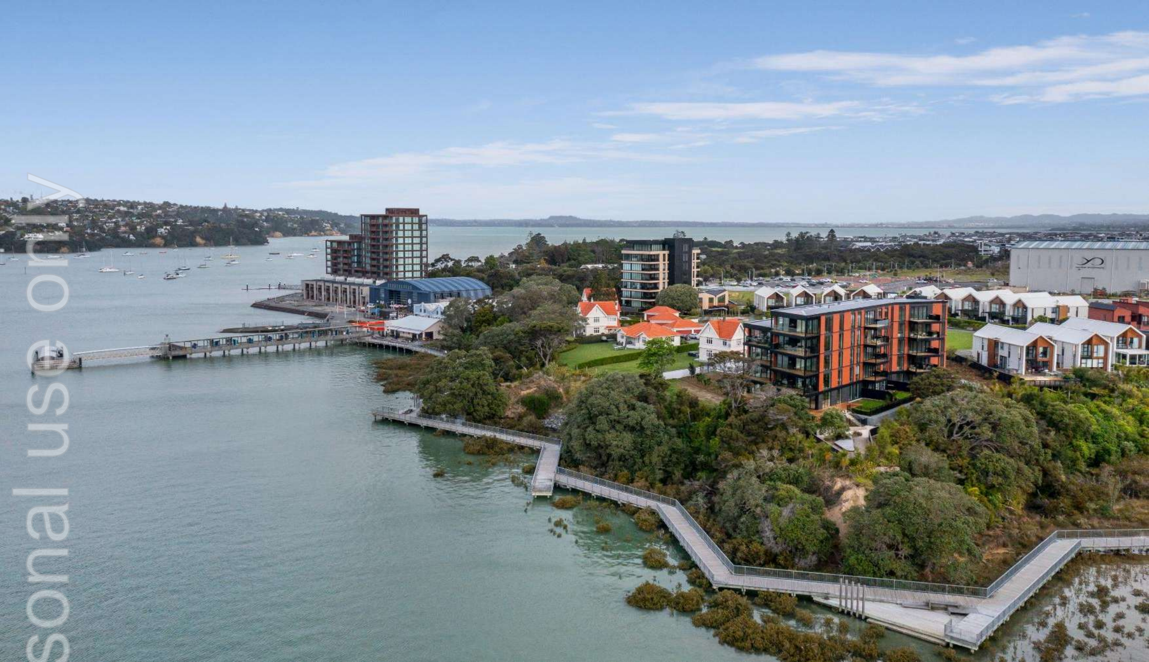
Jimmy's Point, Launch Bay Hobsonville Point
