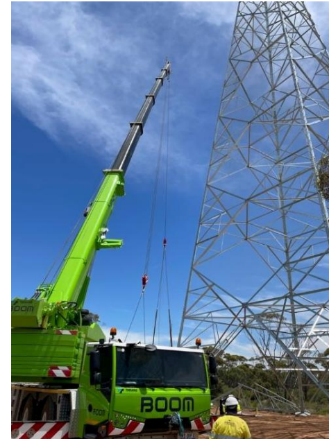
Energy Connect Transmission Project NSW 700km SA to Wagga Wagga Cranes 60t to 150t
