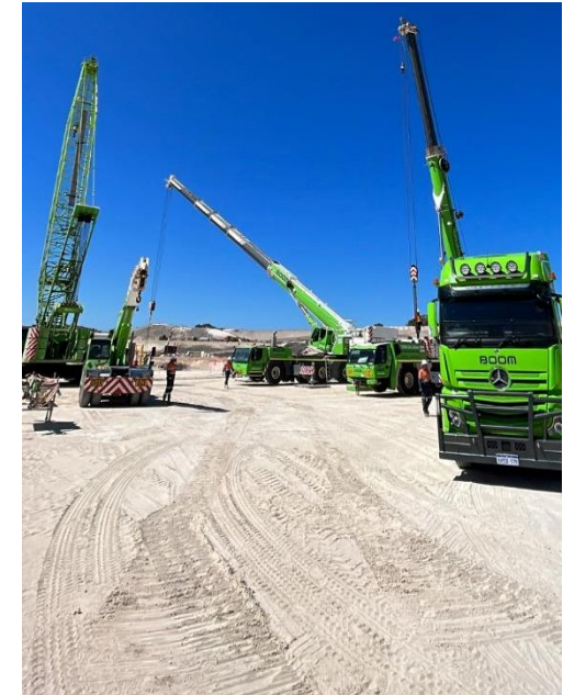
Alkimos Seawater Desalination Plant WA Alkimos, Northern Perth Cranes 150t, 250t & 200t Crawler
