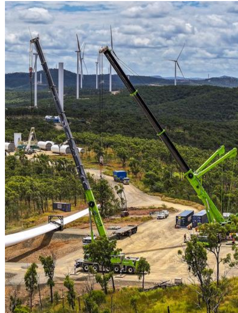
Clarke Creek Wind Farm Northern QLD Turbine construction project 250t & 500t All Terrains
