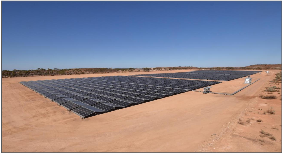
Mt Magnet Solar Farm – February 2025
