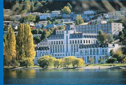
Rydges Queenstown QT conversion
