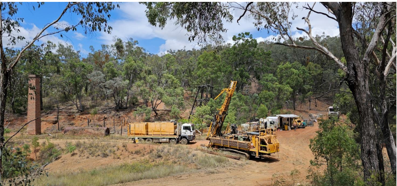
Figure 1: Drilling Equipment located next to the old Gulf Creek Copper Mine headframe and smelter stack
