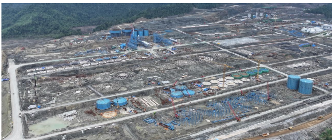
ENC HPAL construction progressing well
