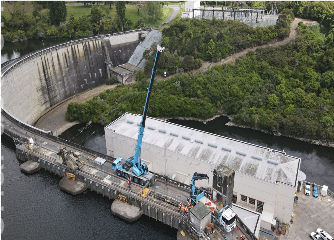
Karāpiro head gate installation
