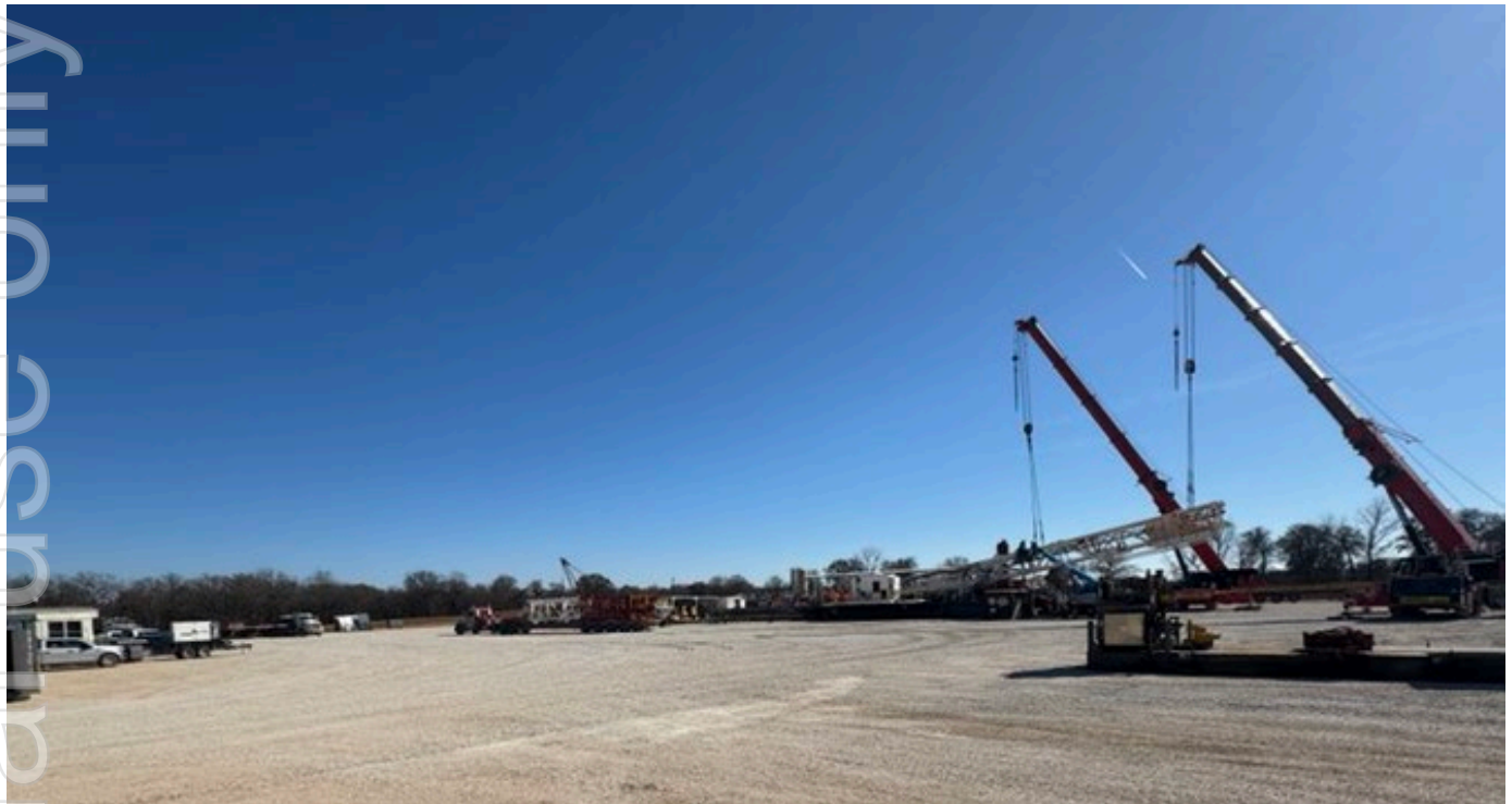
Figure 1. Rigging up Kenai Rig 19 on the Bruins pad in Carter County, Oklahoma.
