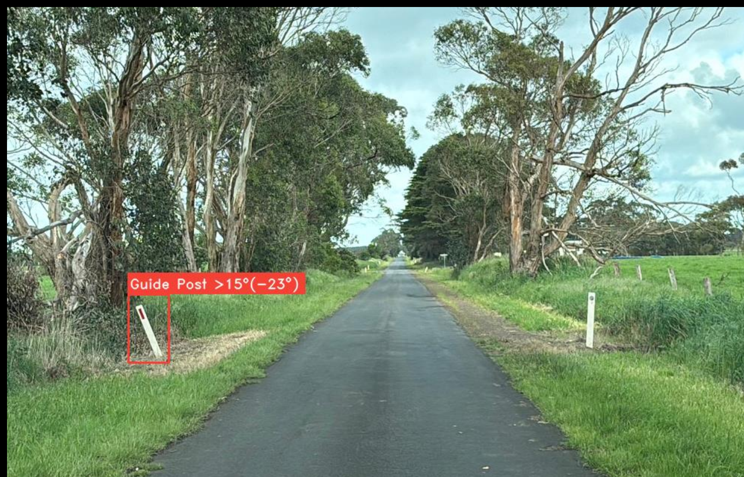
Detection for leaning guide post defects
