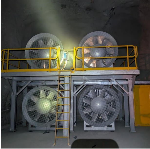
Primary fan installation
