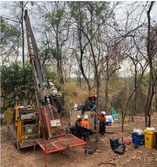
Figure 2: Reverse Circulation (“RC”) and Diamond Drill (“DD”) rigs drilling at Chatree SE Complex.
