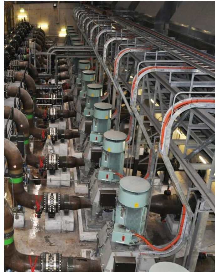
Desalination plants have many large pumps moving a highly corrosive liquid at high-pressure.
