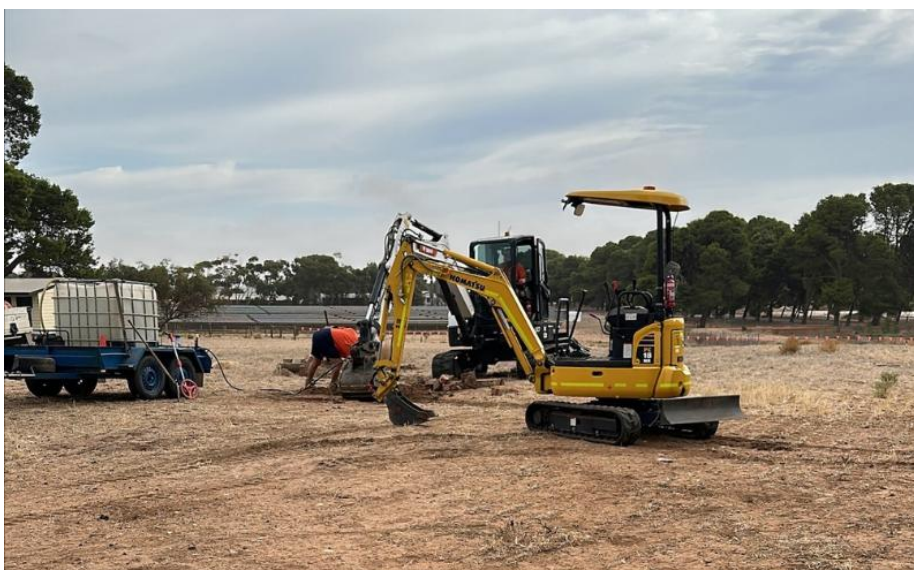
Figure 1: Site preparation activities, Roseworthy, South Australia
