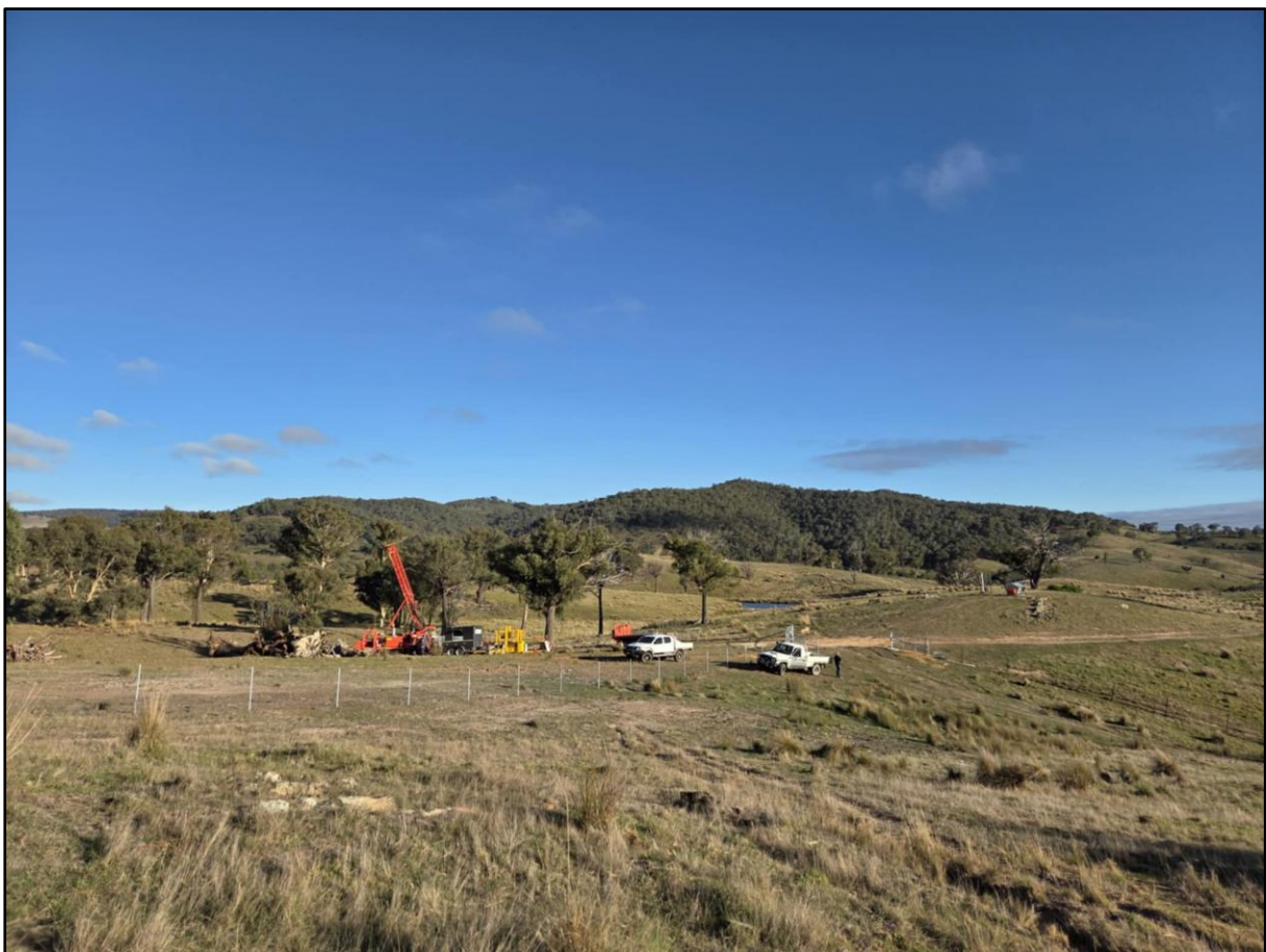
Figure 1: Drill rig set up at the Picker Prospect.
