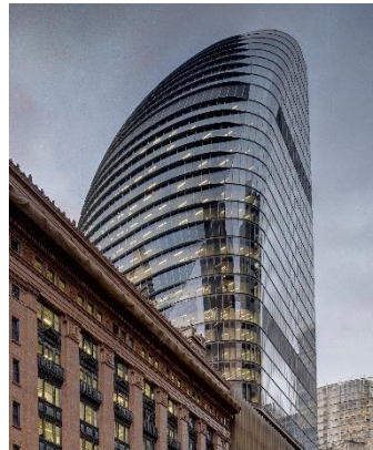
Macquarie's new global headquarters at 1 Elizabeth Street
