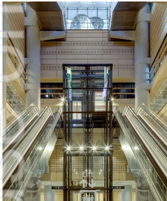
Martin Place metro station as part of Australia's largest public transport project
