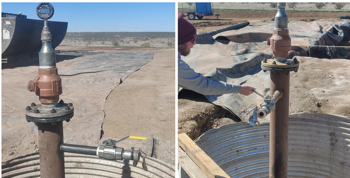
Well-head testing at Jackson 31 well, Galactica Project
