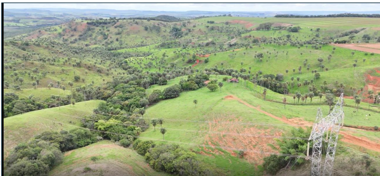
Figure 3: View to north, at North of the Tiros Central block with high voltage power line in the foreground
