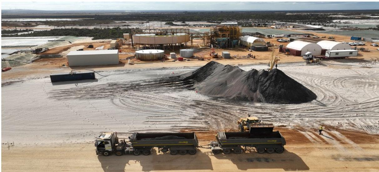
Photo 1 – Atlas HMC first transport to Geraldton storage – 12 March 2025
