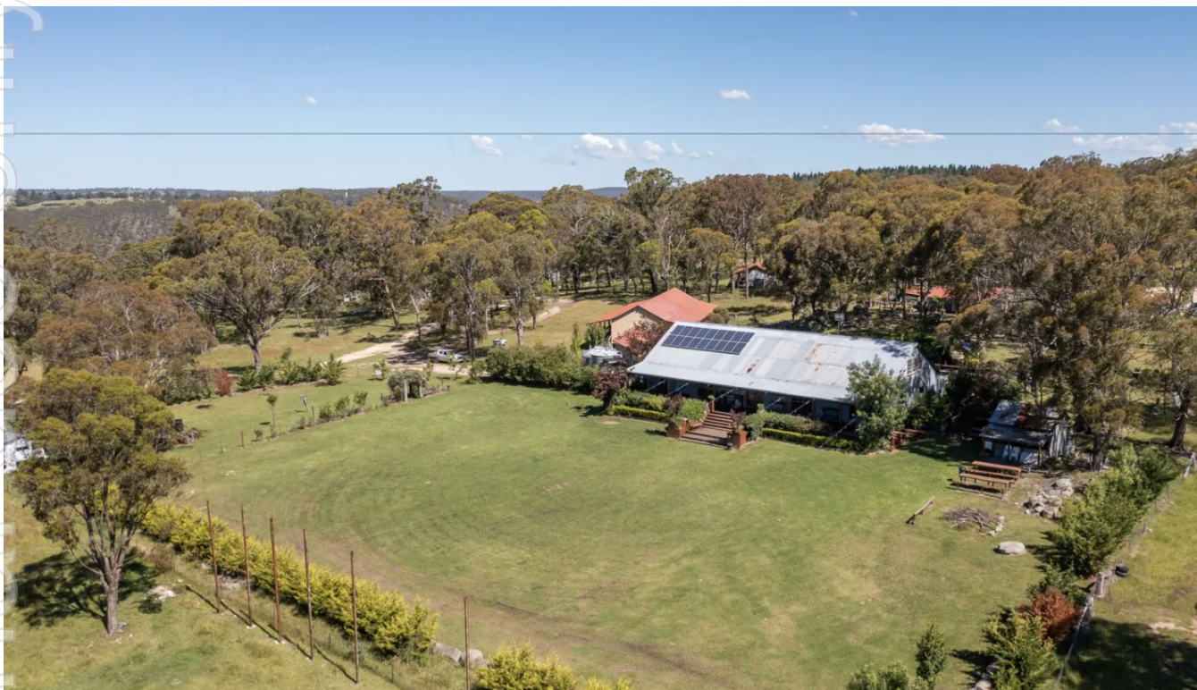
Figure 1. Aerial view of Echidna Gully Dining facility (foreground) and accommodation (rear)
