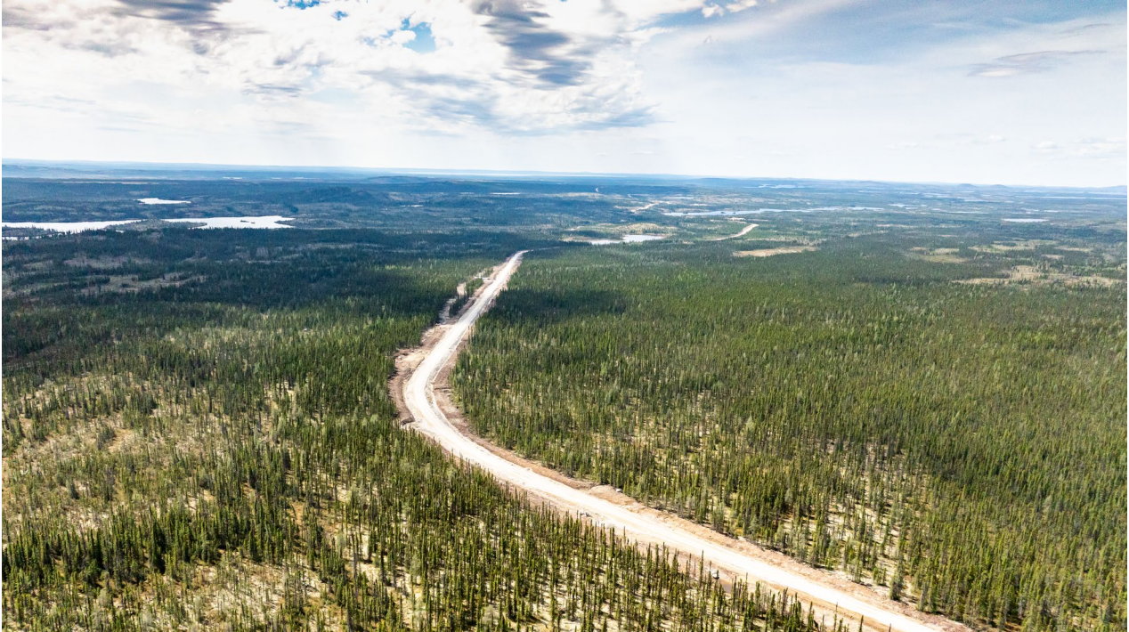
Figure 2: A portion of the all-season road (~20 km in length) built by the Company, extending from the all-season Trans-Taiga Road to the CV5 Spodumene Pegmatite.
