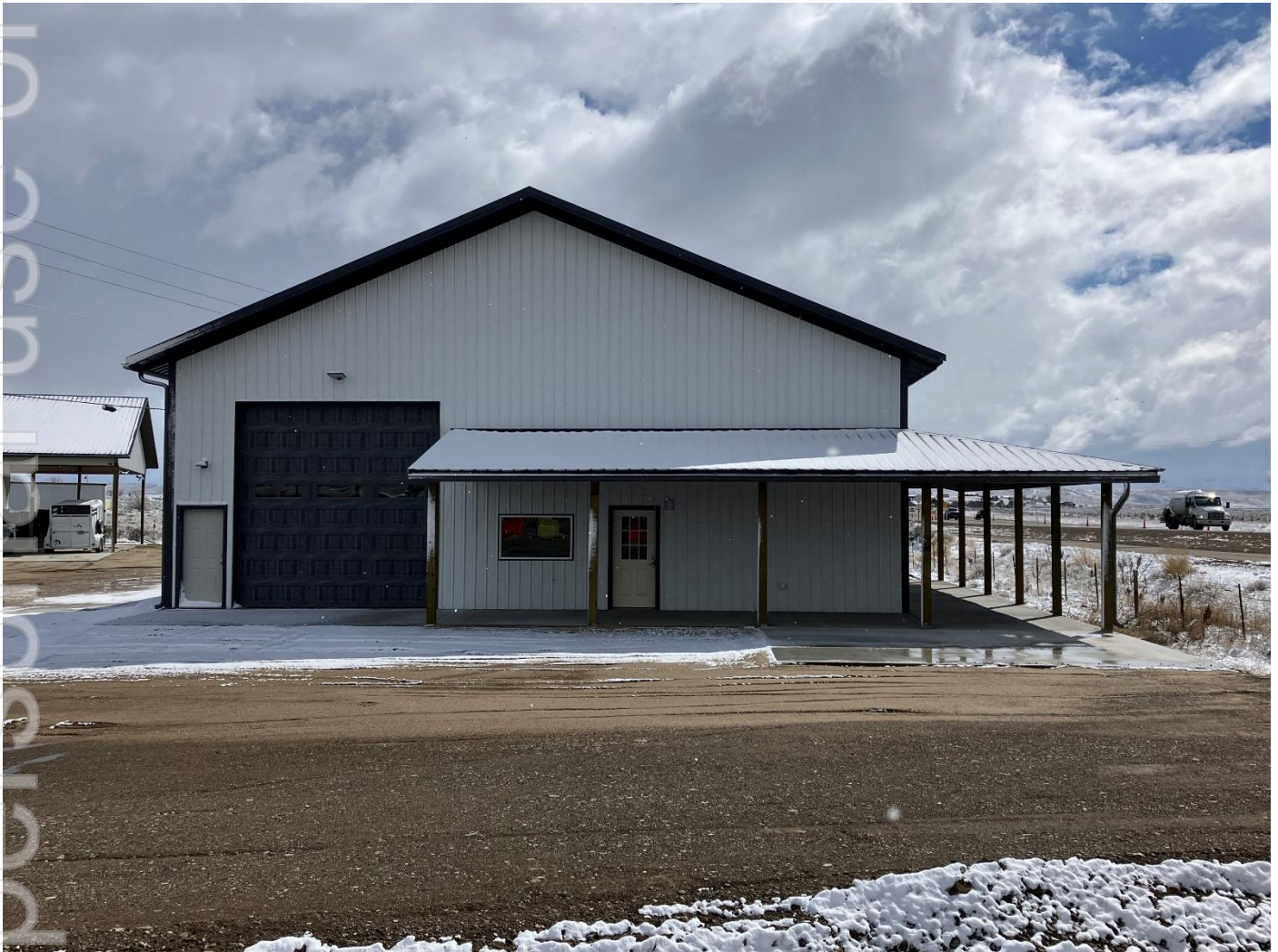
Figure 1 – Sun Silver's core processing facility / exploration hub located in Elko, Nevada.
