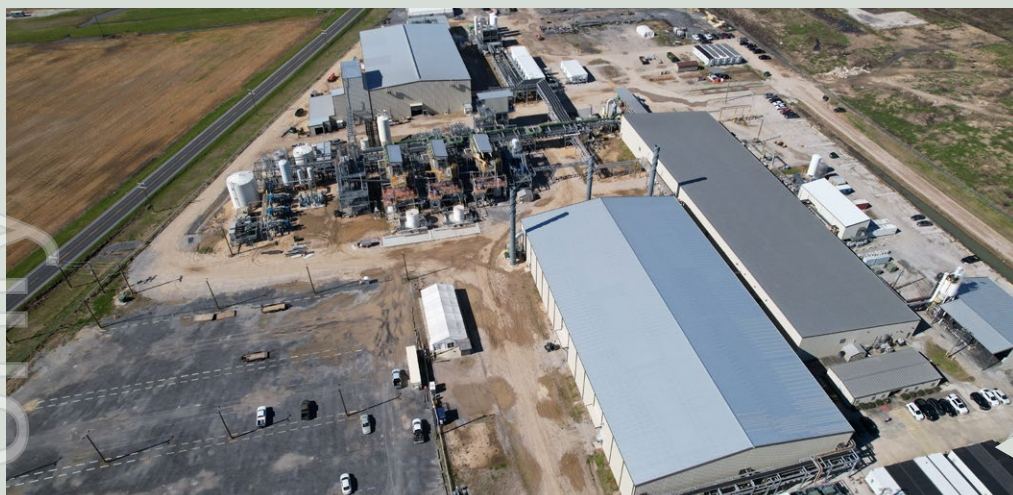
Vidalia AAM facility
