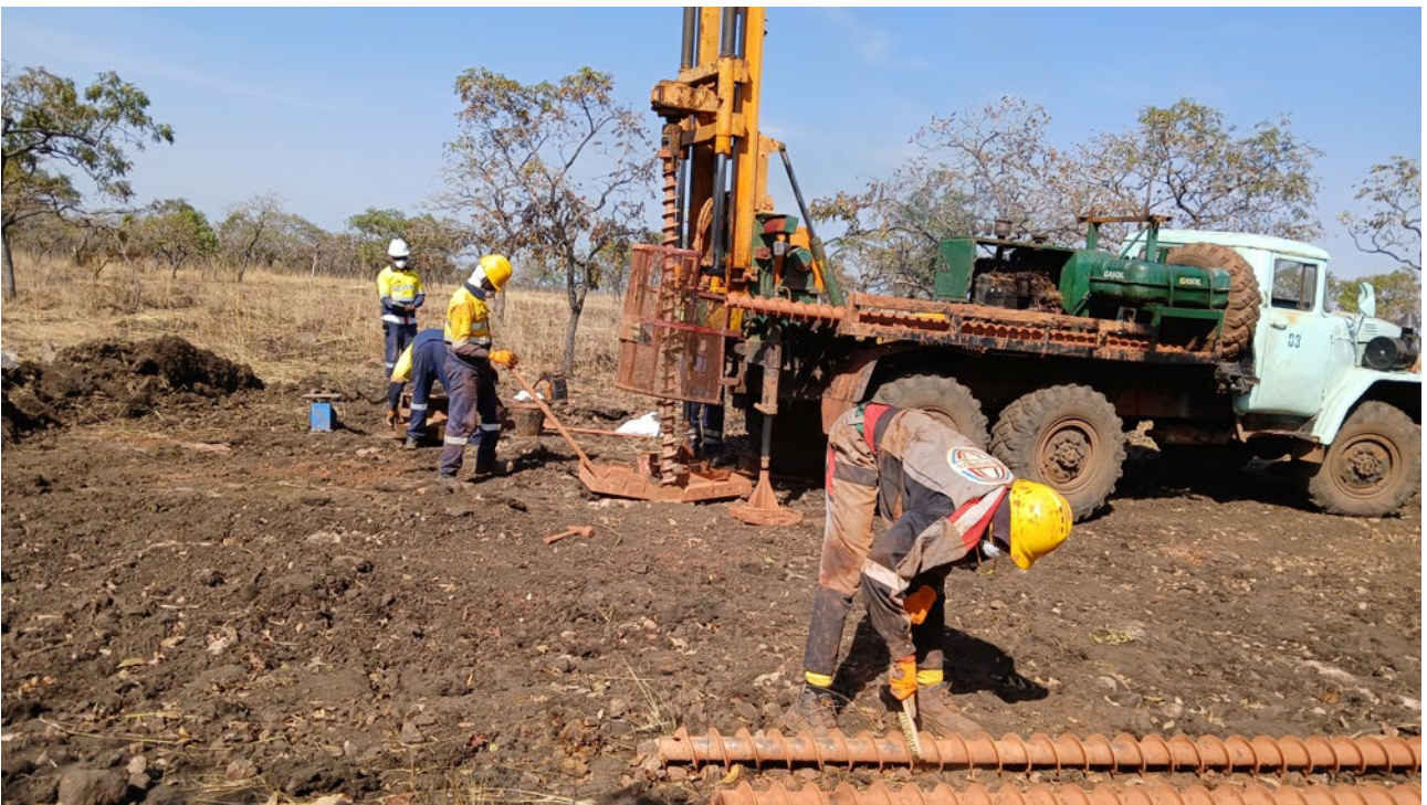
Figure 6. Geoprospects auger rig technician cleaning auger flight to prevent sample contamination
