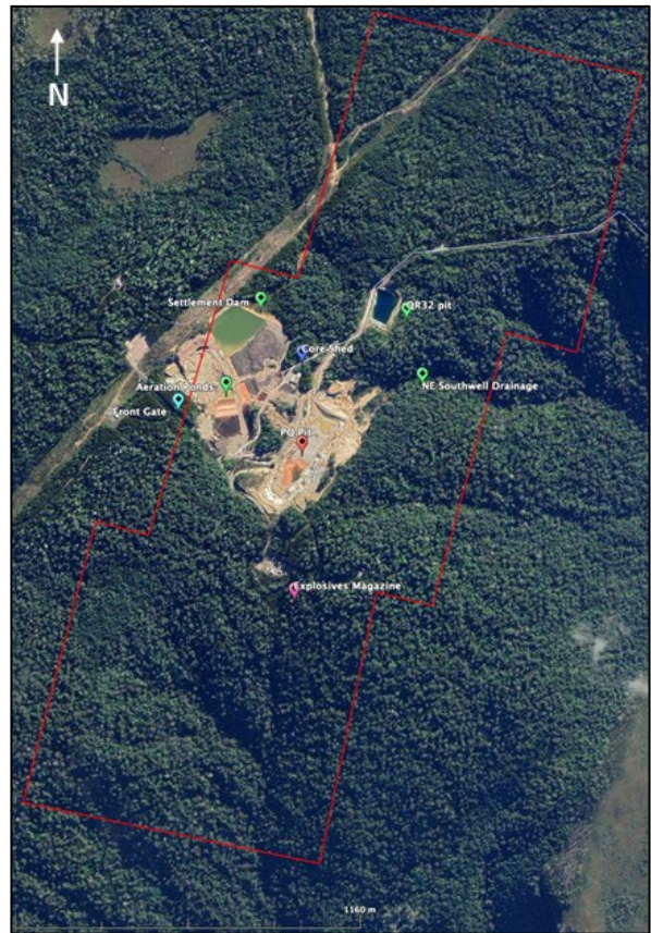
Figure 2 Que River aerial view (2021 regional grid)
