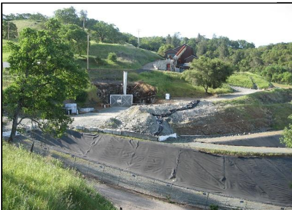
Portal and Processing Plant
