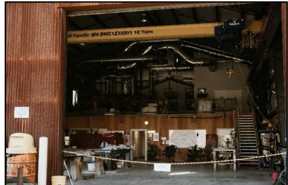
Workshop With 10 Ton Crane
