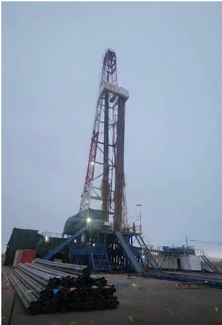
Figure 2: DWK Drill Rig at the Red Lake Gas Field in the South Gobi
