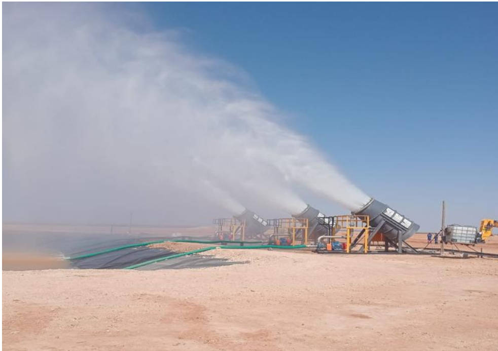
Photo 1: Water evaporation on site at PCZM.
