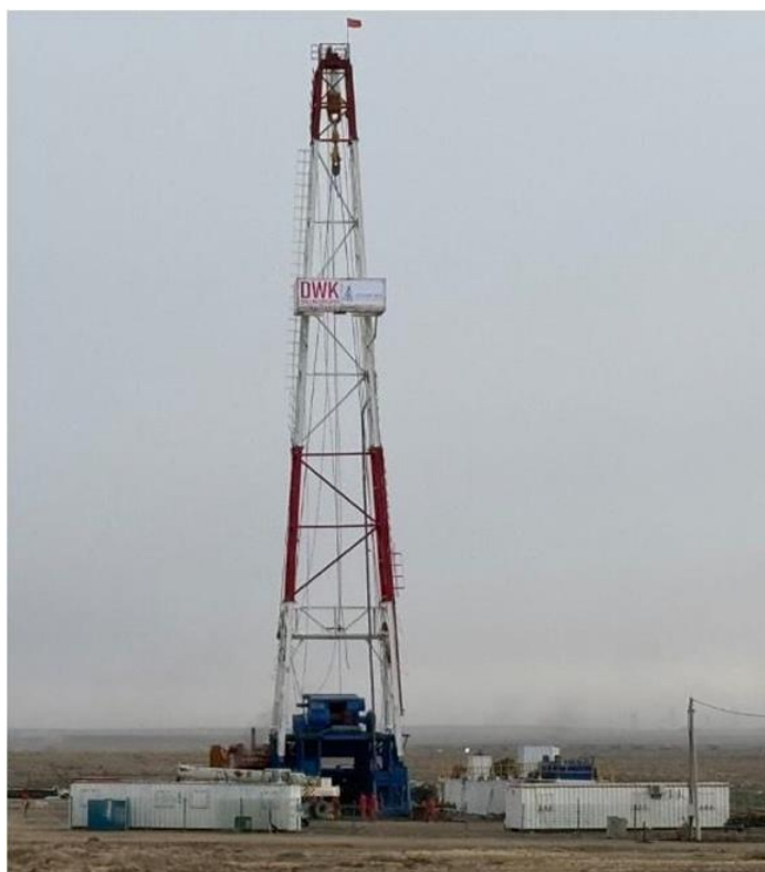
Figure 6: DWK rig in place for Jade's lateral well program
