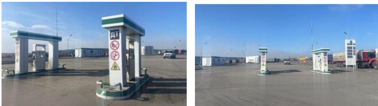
Figure 2: UBM's LNG Fuelling Station at Tavan Tolgoi
