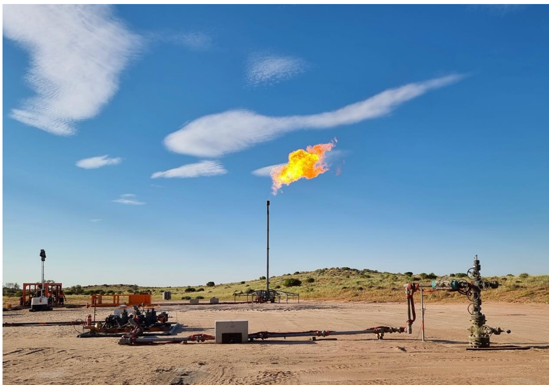
Figure 3: Gas flare from Kiwi-1 wellsite at 1.7 mmcf/d
