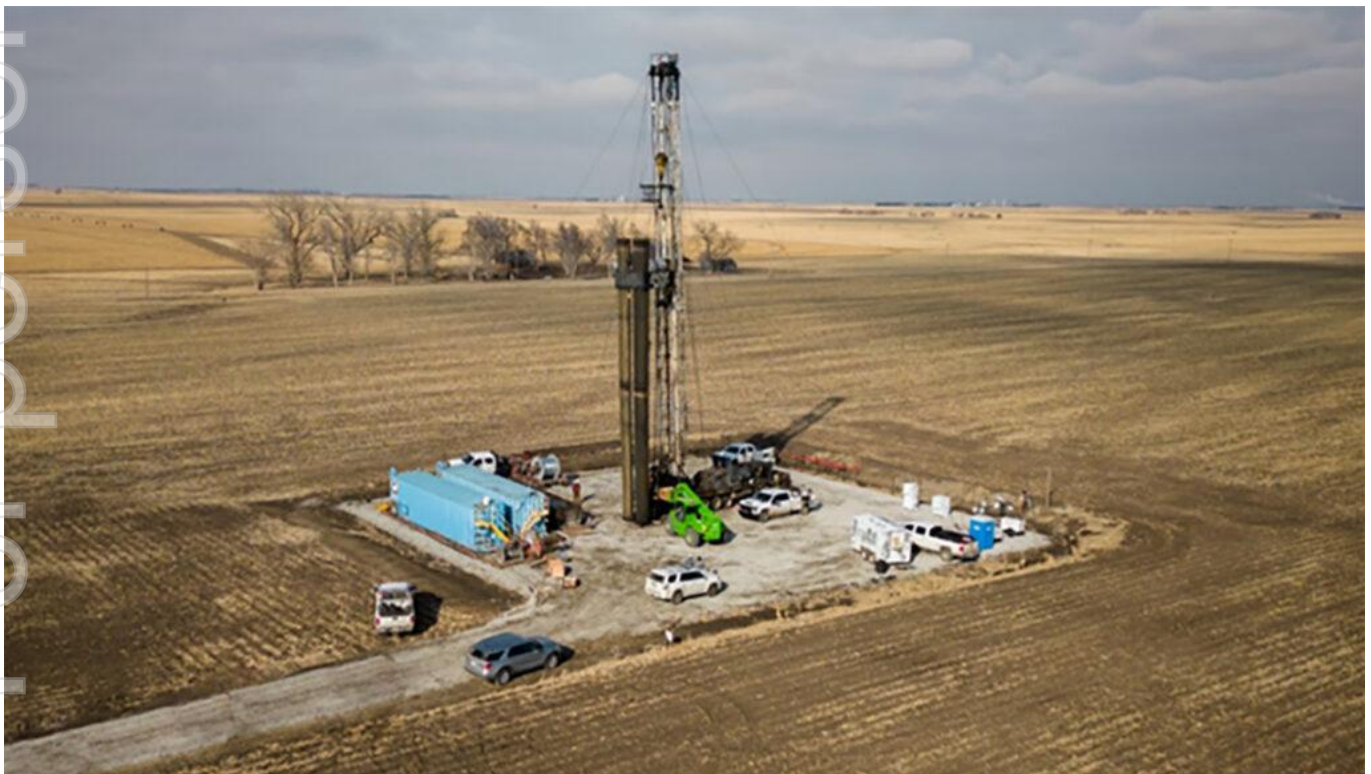
Figure 6. Wildcat well specifically targeting white hydrogen (Hoarty NE3) in Geneva, Nebraska.
