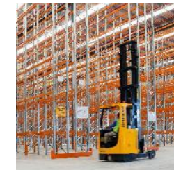
Ingleburn Logistics Park
