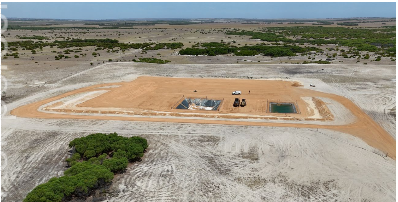
Figure 1: Becos-1 well pad completed
