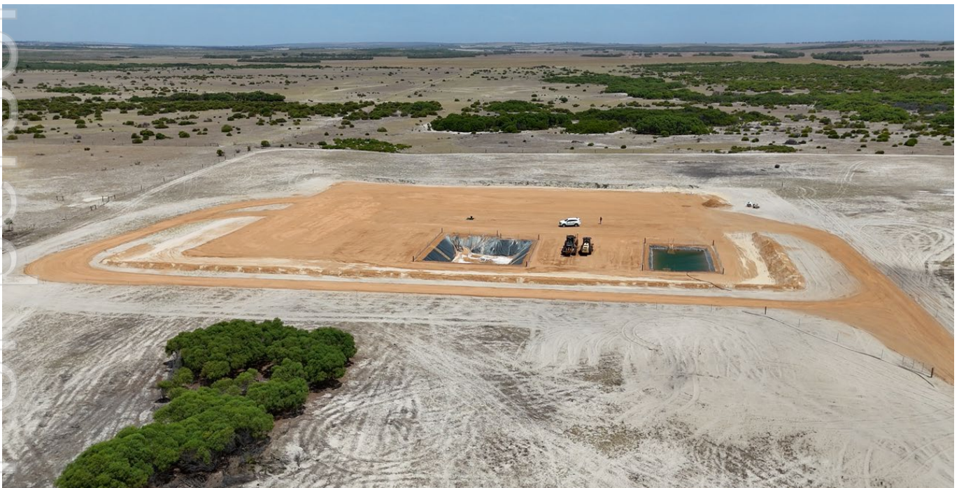
Figure 1: Becos-1 well pad completed
