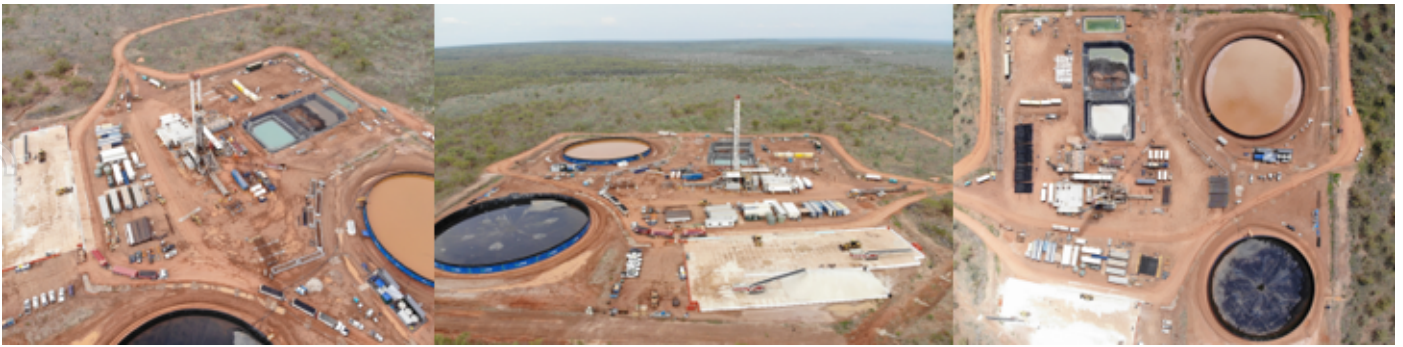
Drone photos of C-5H
