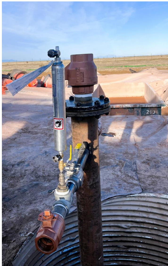
Well-head testing at Jackson 4 well, Galactica Project
