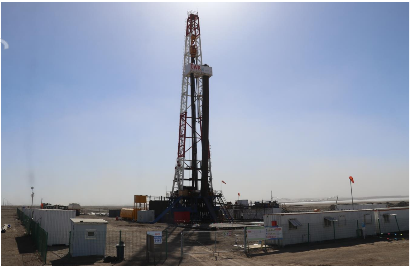
Figure 1: DWK Drill Rig Commencing Second Lateral Production Well at Red Lake
