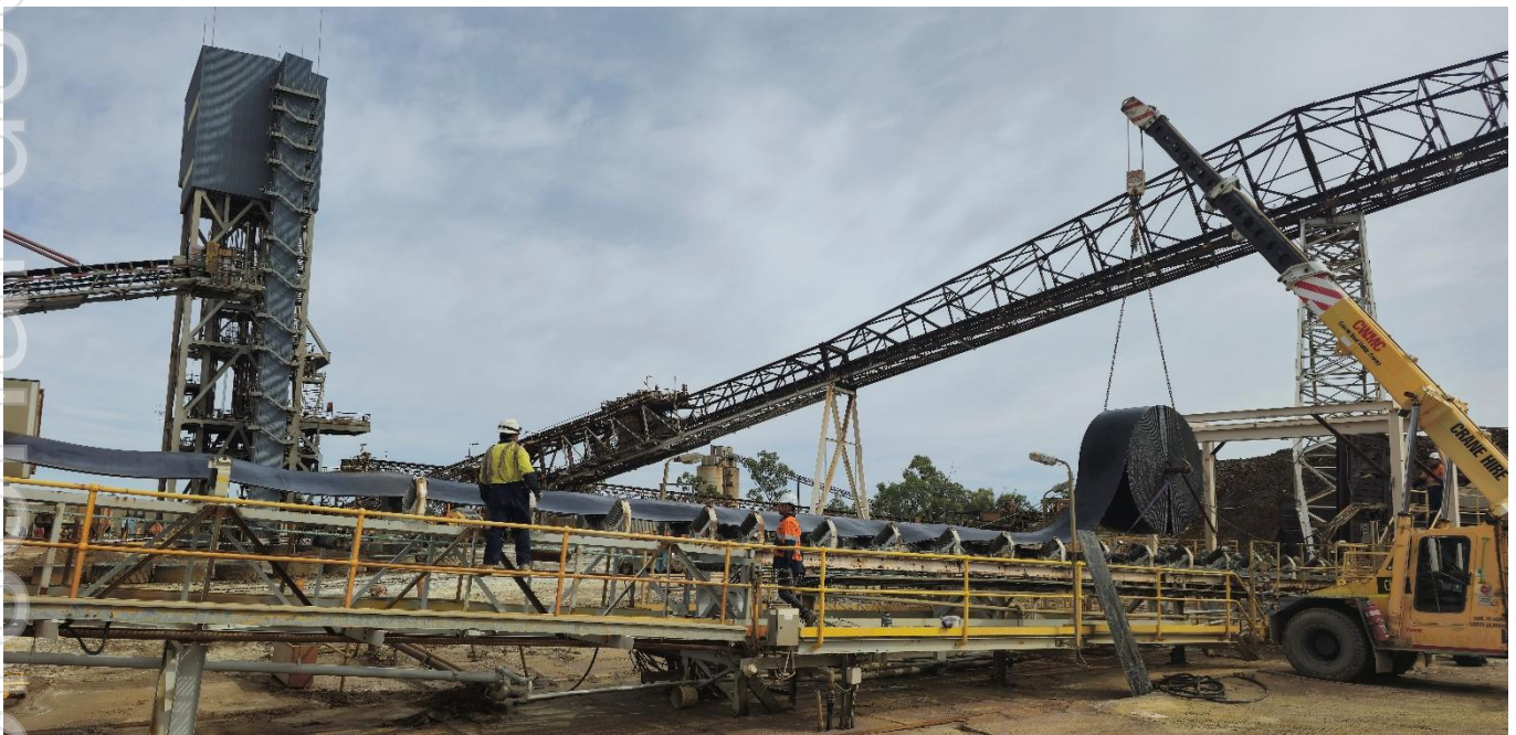
Figure 4: Replacement of mill feed conveyor.
