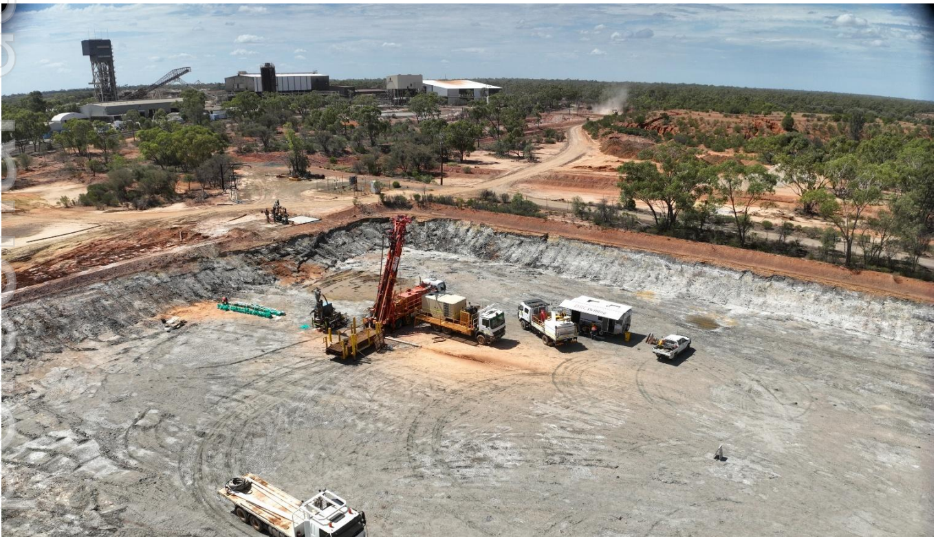
Figure 5: Drilling of southern extension within the recently cleaned Process Water Pond.
