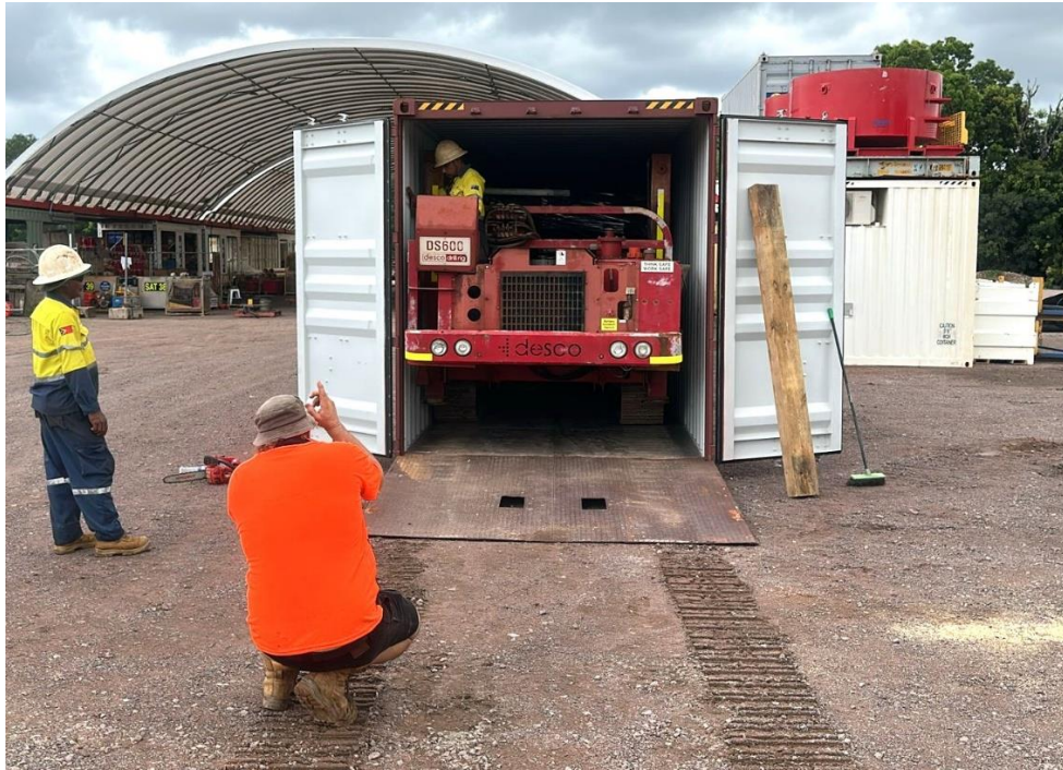
Figure 3: Rod slew carrier being loaded into one of four 40 foot sea containers ready to transport by ANL to the Dili Port
