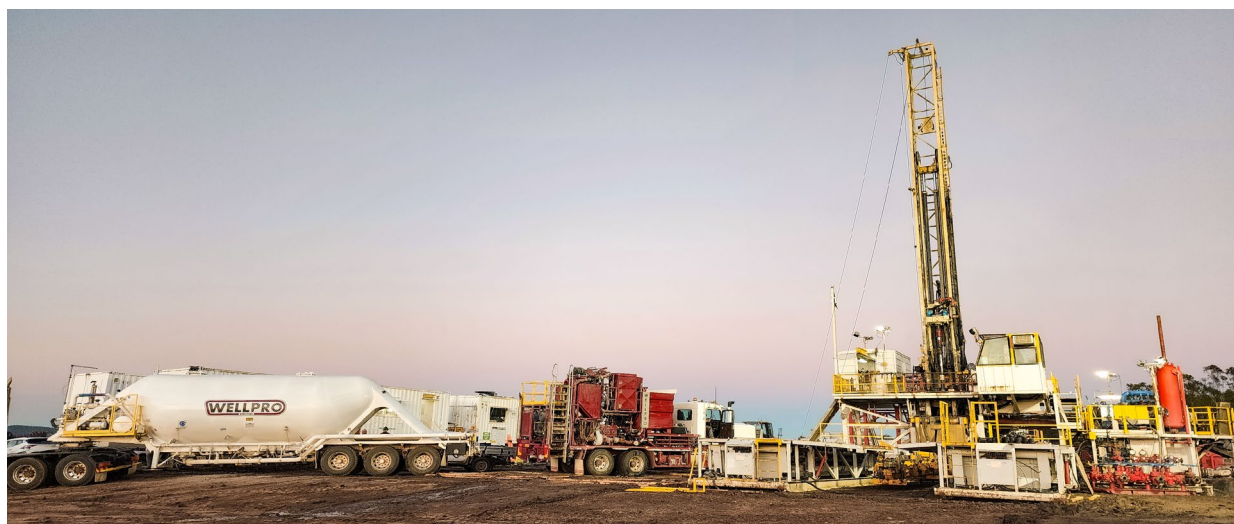
Picture 2: Cementing operations. Photo credits: Molly McEwin
