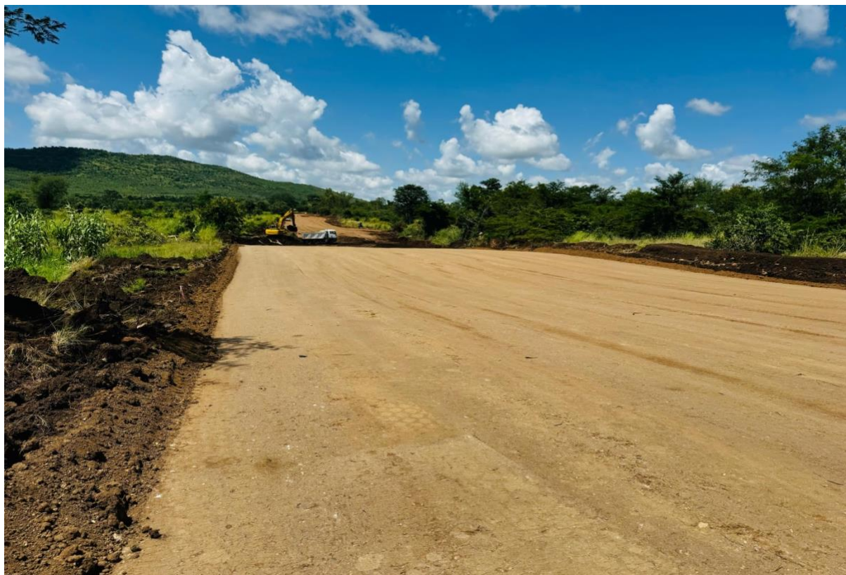
Figure 3 - Access Road construction well underway to the Kangankunde Project.
