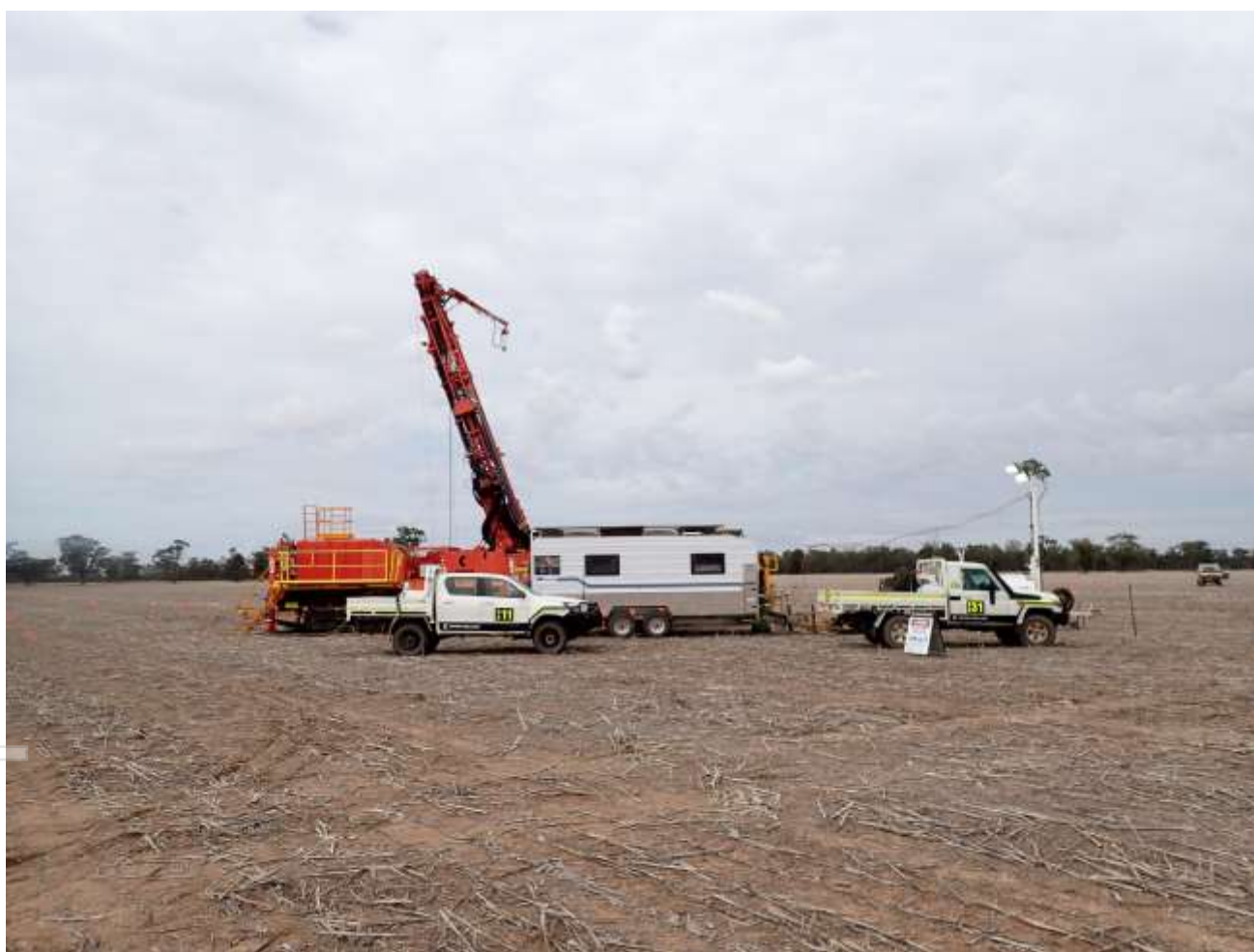
Figure 1. Rig onsite at Calais.
