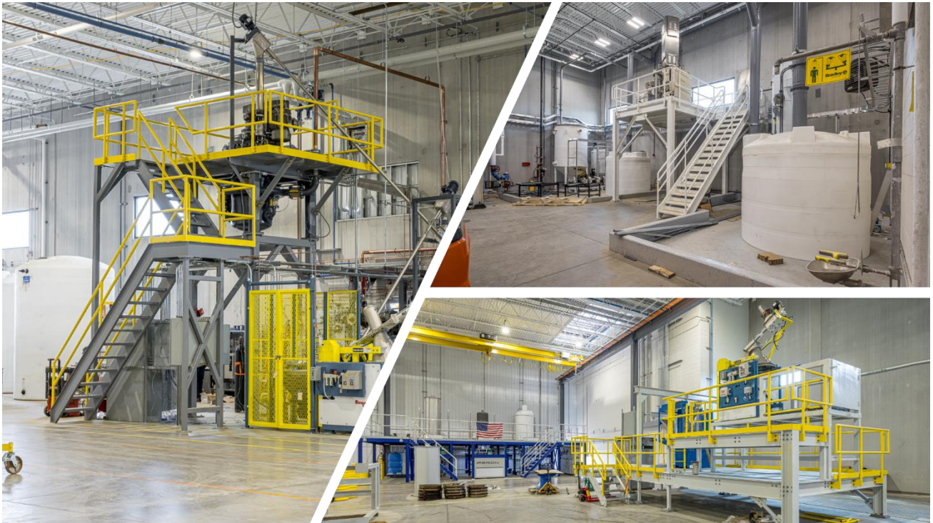
Figure 2: Ancillary Equipment and Utilities Installation
