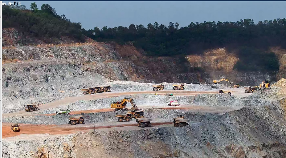
← Pushing back the A Pit West towards A North
