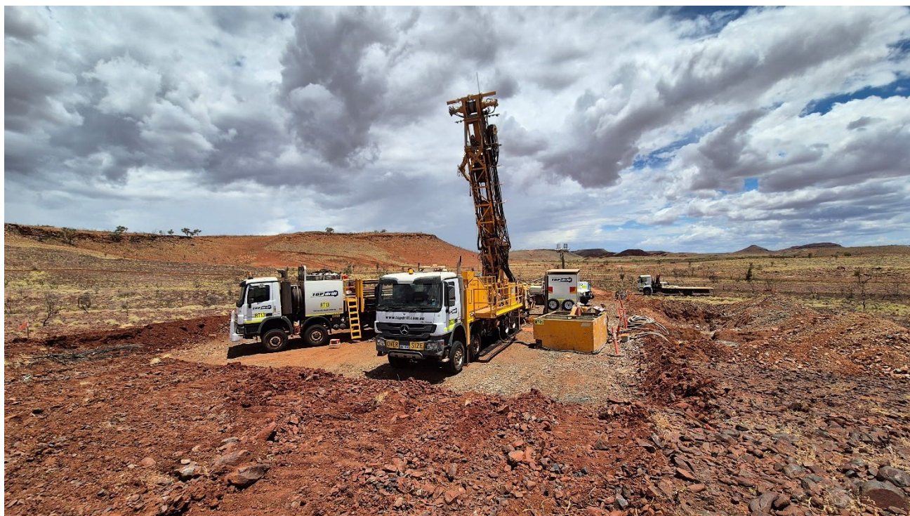
Figure 1: Drilling the Shelby target at the Whundo cluster of VMS style Cu-Zn deposits
