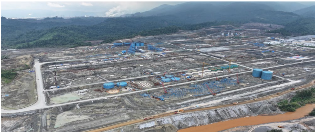
ENC HPAL construction progressing well
