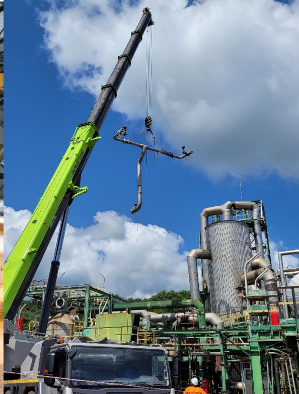
Figure 4: Acid plant refurbishment
