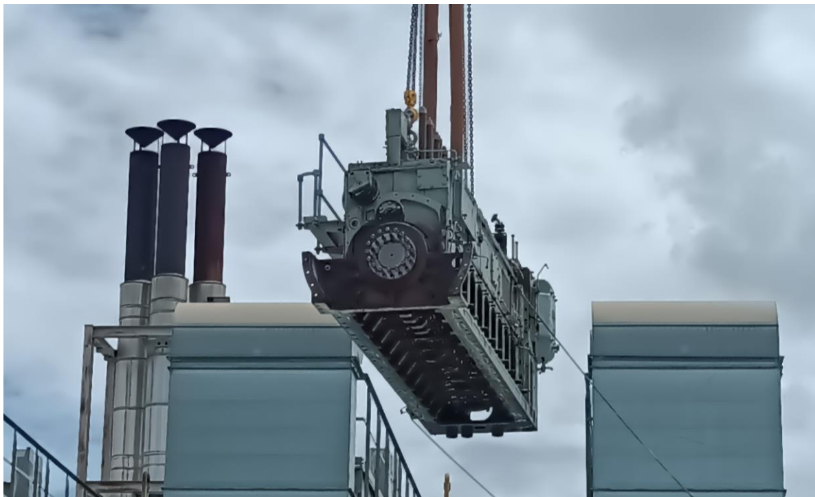
Figure 2: Hyundai diesel generator lift during power station overhaul
