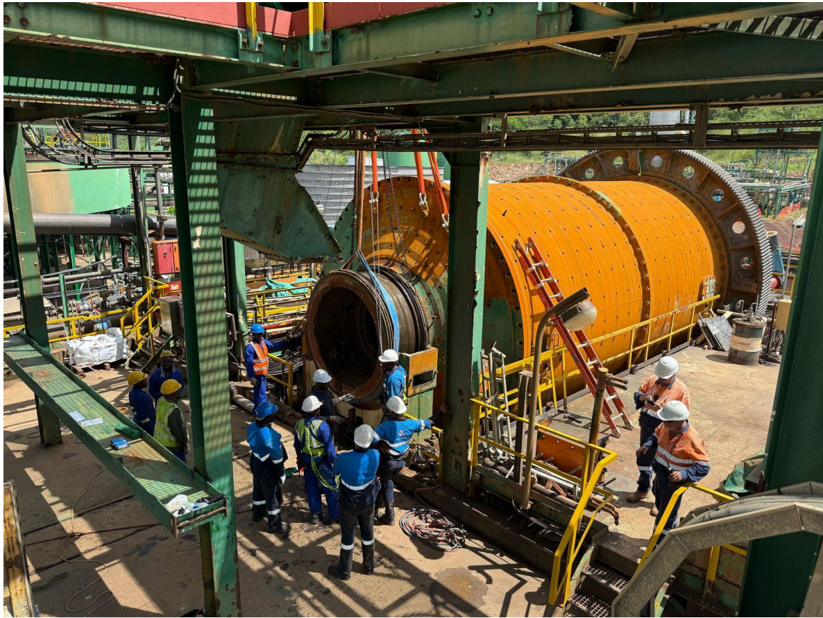
Figure 1: Mill refurbishment activity
