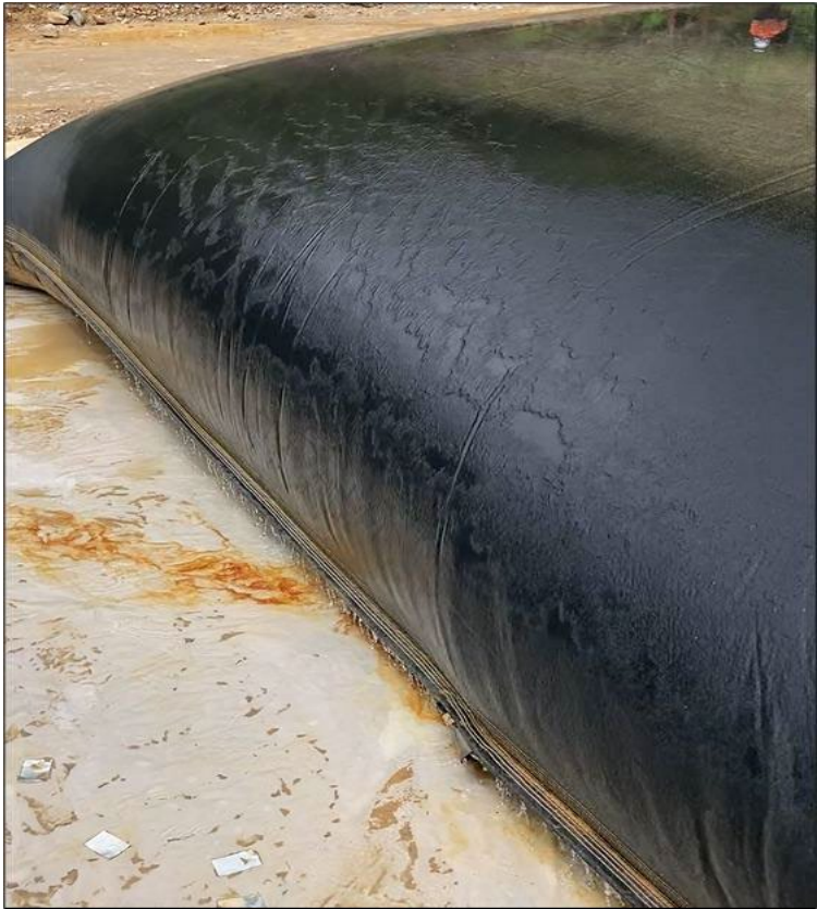
Interim Tailings Geotube
