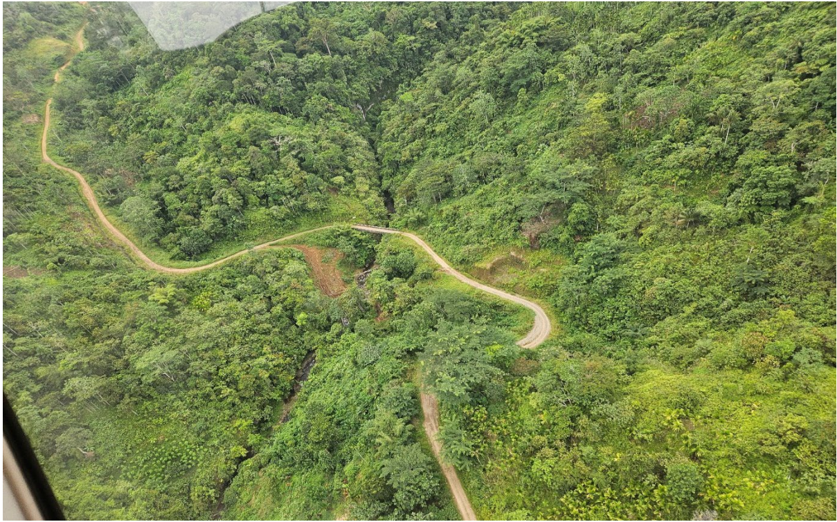
New Tolukuma Access Road
