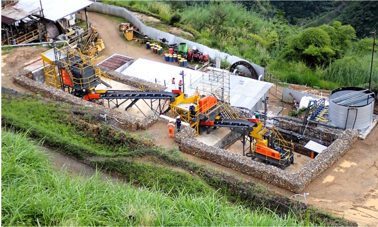
APT Modular Gravity Plant installed, December 2024
